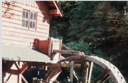
Our "once and future" flume was/will be a wooden chute supported by chains.
